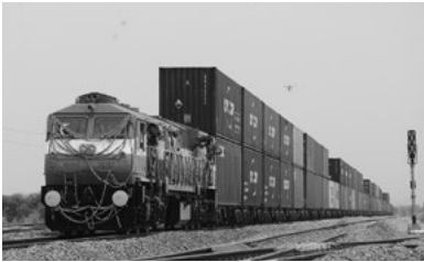
Delhi–Mumbai dedicated freight corridor project (Trial run during partial operations of the track)
