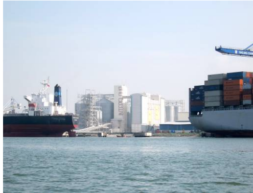
Interflour Vietnam's specialized port facilities for grains
