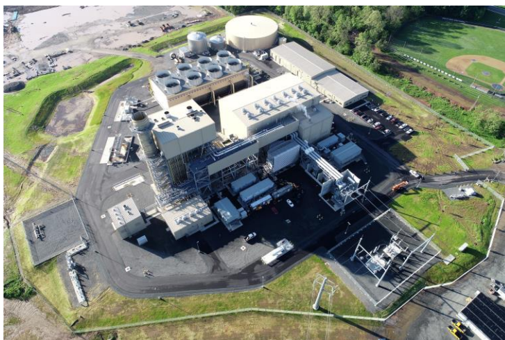
[Power Plant Facility]
