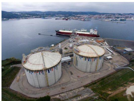
[Overhead view of the Mugardos LNG Terminal]
