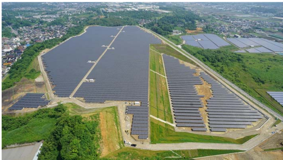
[Iizuka Kami-Mio Solar Power Plant]
