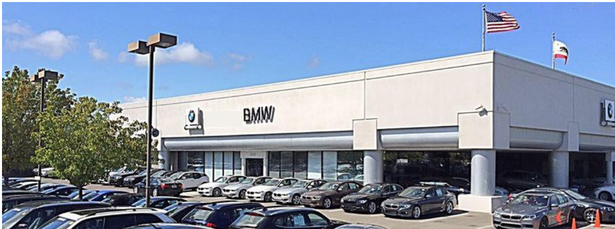
BMW of San Rafael (formerly Sonnen BMW) Center Facility
