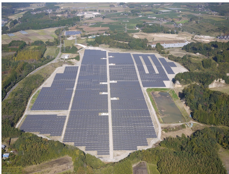
[Overhead View of Kuma Nishikimachi Solar Power Plant]
