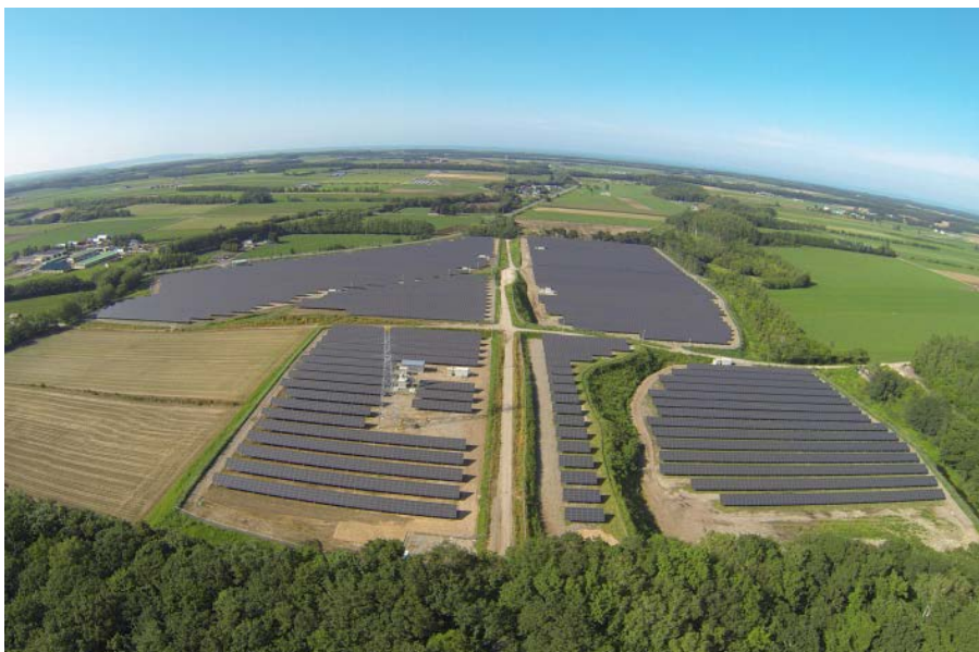
[Overhead View of Koshimizu Solar Power Plant]
