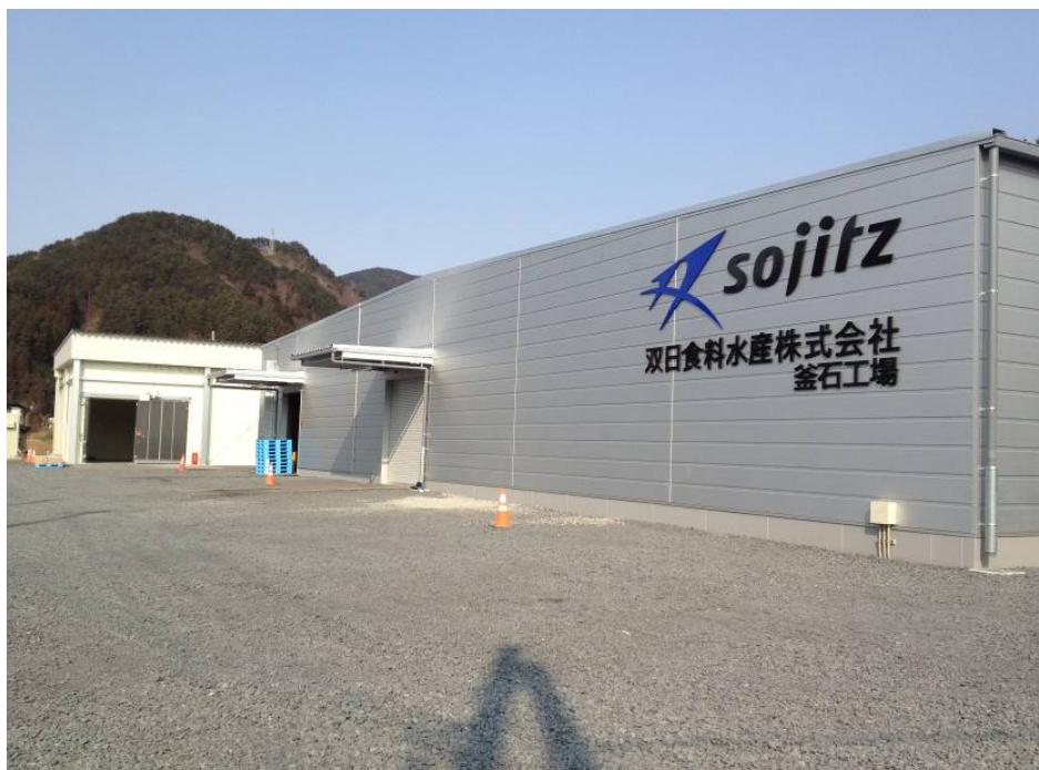
The completed new plant
