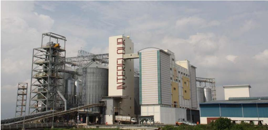
IFV's milling plant, silos, grain elevator, and cargo conveyor
