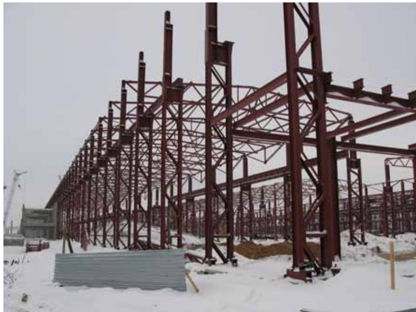
[Railway Freight Car Production Plant under construction in Kanash]
