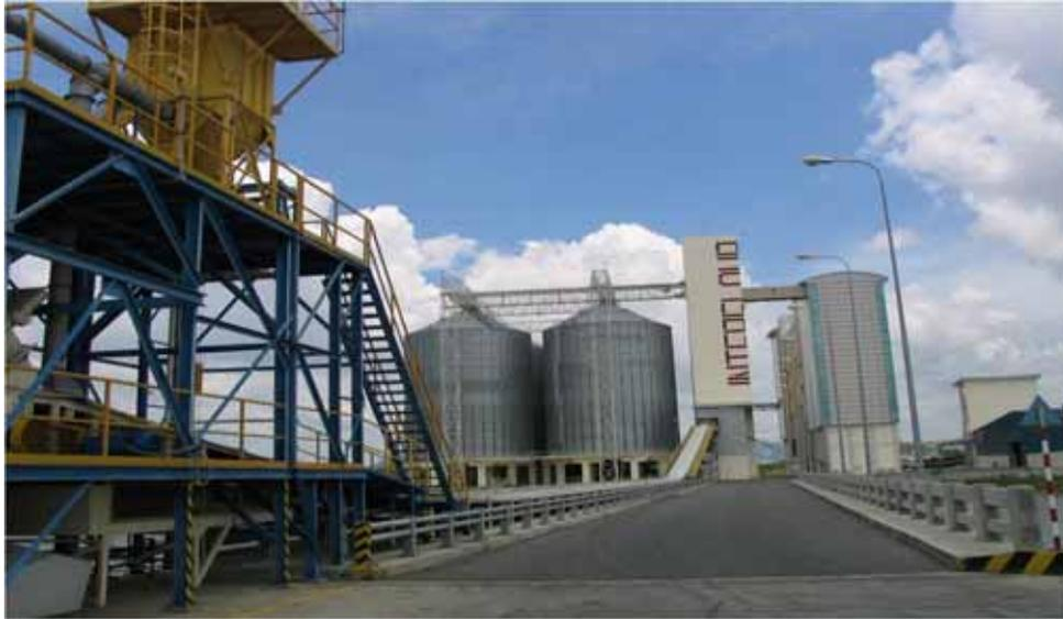
IFV's milling plant, silo, grain elevator and cargo conveyor
