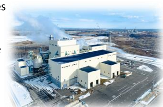
Yufutsu Biomass Power Plant
