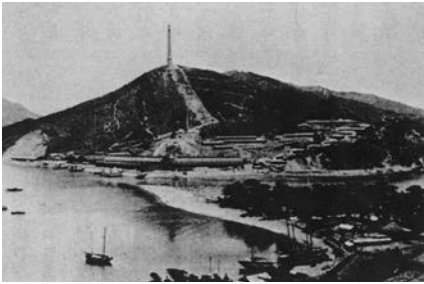
The 72-meter chimney (while in operation)
