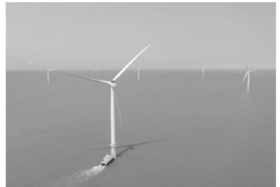
Sojitz entered Taiwan's largest offshore wind power project in 2019 (copyright with permission by Yunneng Wind Power Co., Ltd.)
