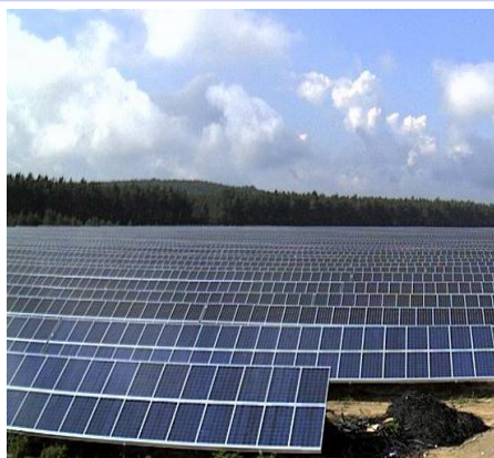
Solar power generating facility in Mixdorf, Germany
