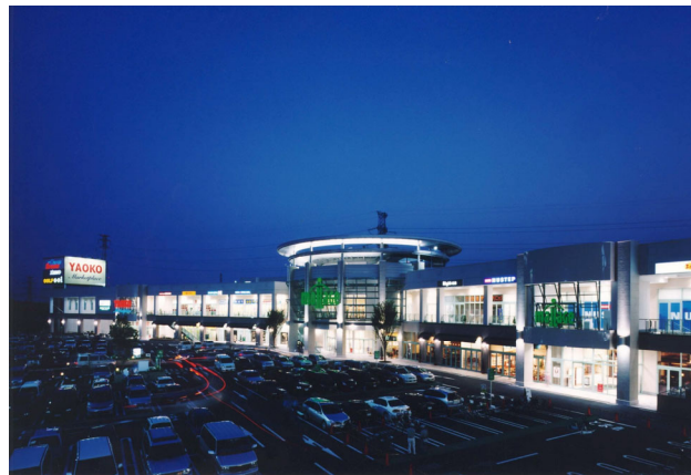
Mallage Kashiwa (exterior)
